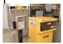
Exit to East Drive. Gate 1
